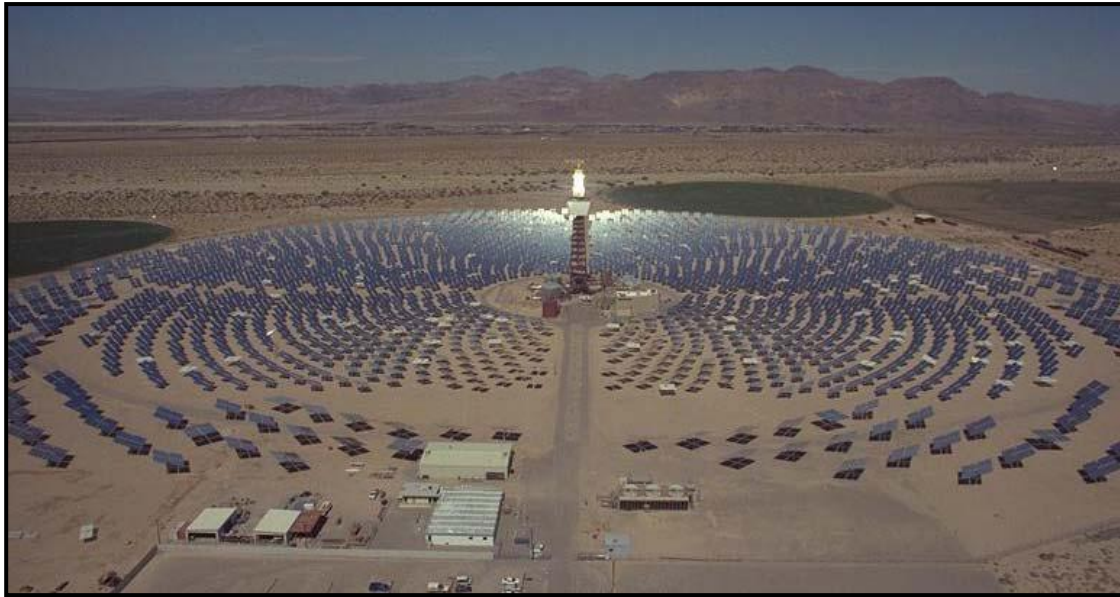
Figure 3.1.5: A 10 MW Solar Farm Project near Barstow, California (Nexant, 2010)
